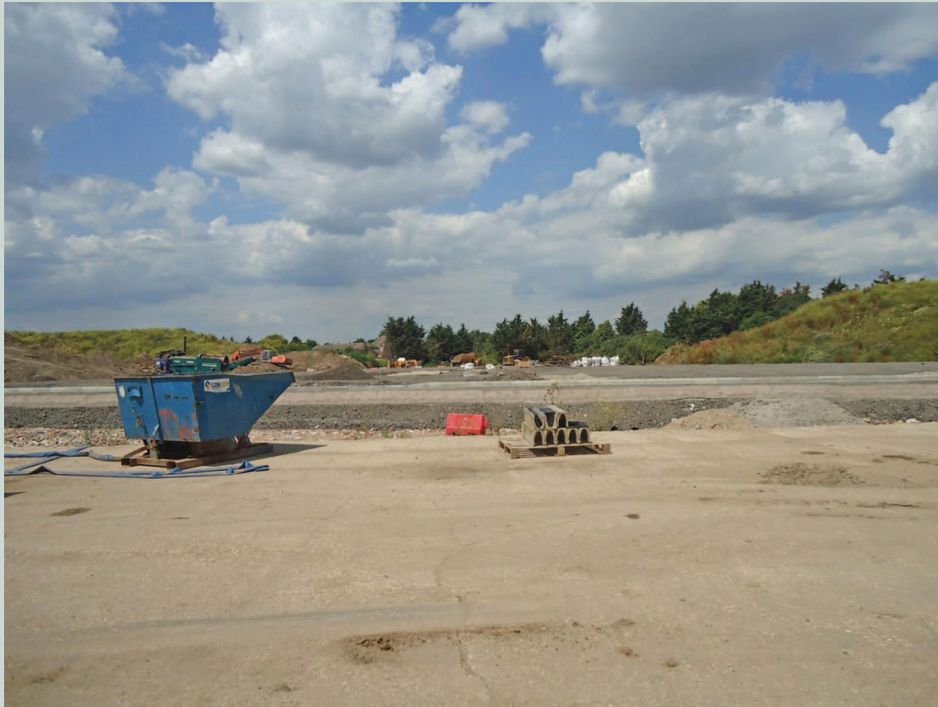
Fig 5 : Existing site operations looking Northwest
