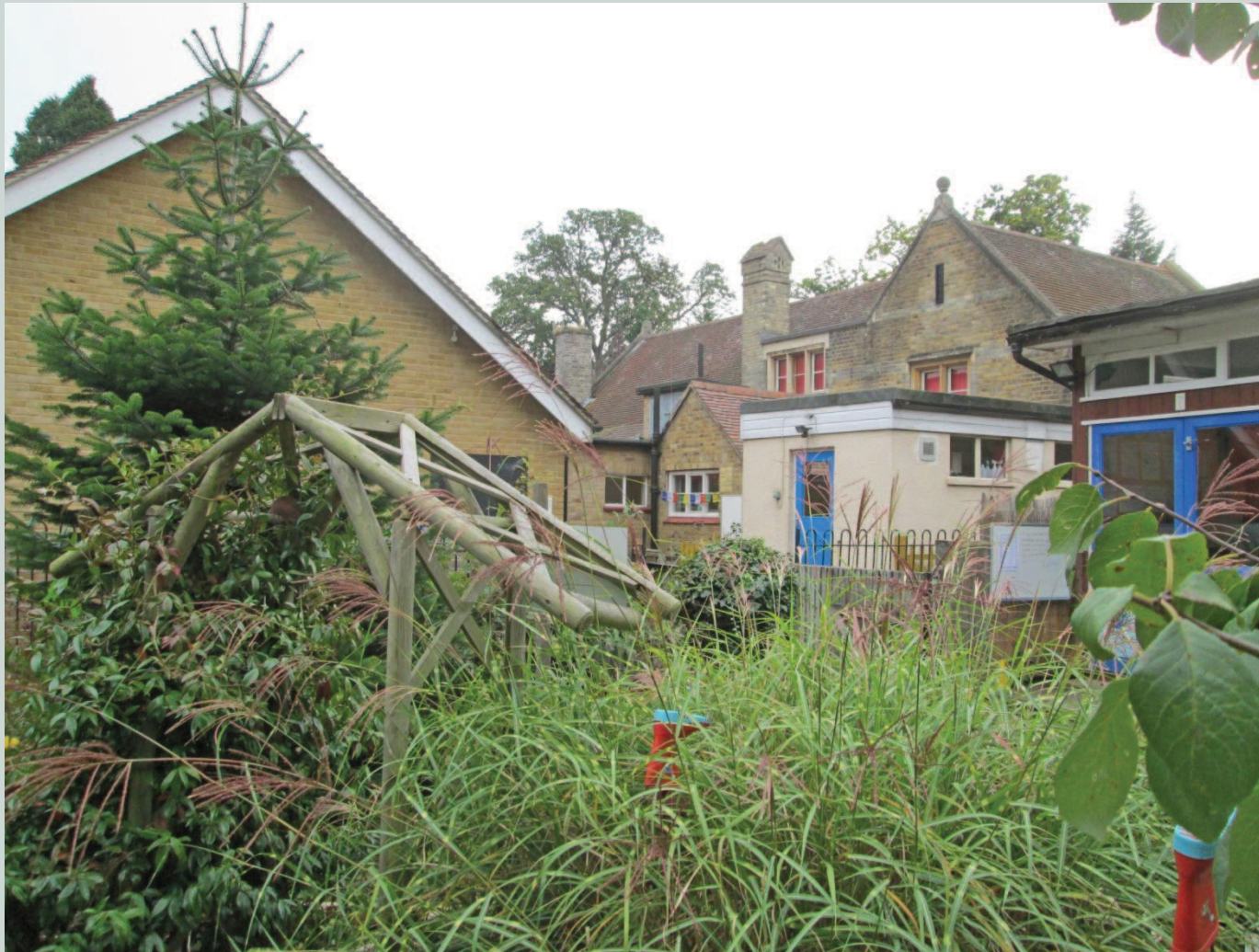
Fig 4 : Existing main building and hall, viewed from rear (north)
