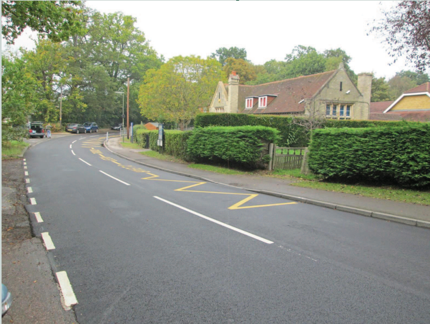
Fig 1 : Existing School Building, with hall behind, viewed from South west across Lyne Lane
