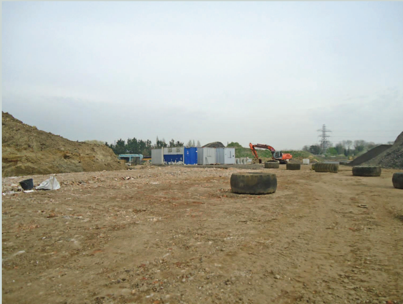
Fig 2 : Existing site operations looking Northeast
