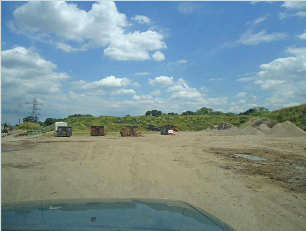
Fig 3 : Existing site operations looking East
